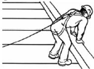
**PR600 system:** The distance of the pivot arms to the leading edge must be no less than 15 feet. The ballast basket must be extended out to a distance of nine feet from the pivot arms. The amount of the weight to be placed into the ballast basket is 500 pounds.
